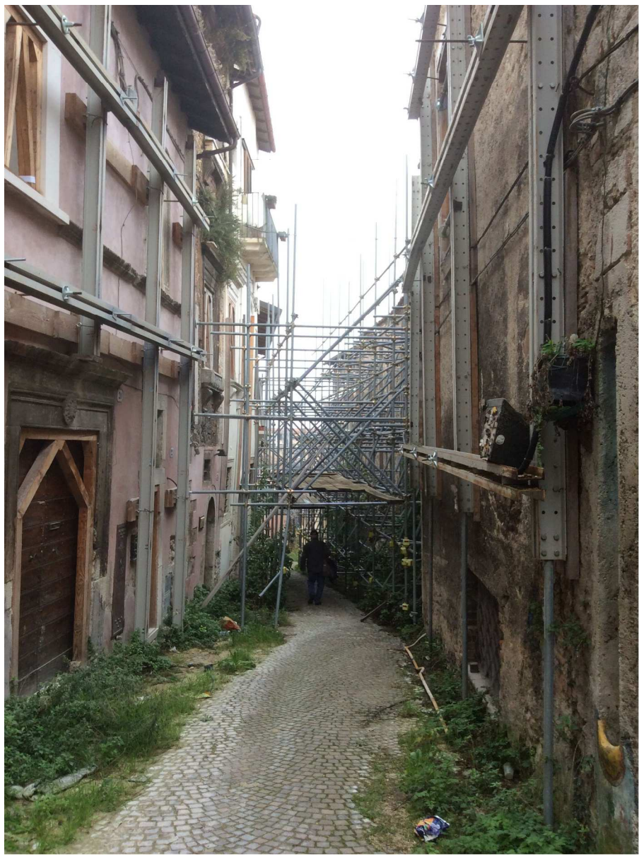
Figure 3. A street in L'Aquila city, October 2016 (photo: author).
