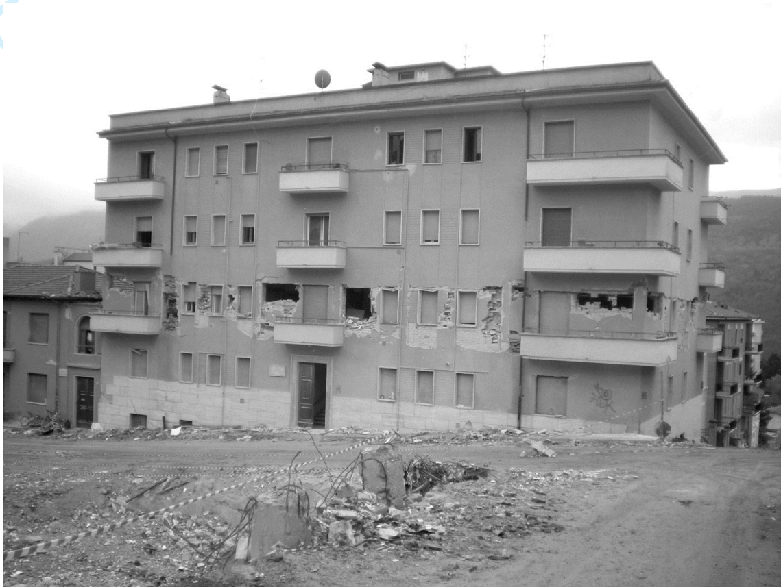
34 35 Figure 2. An example of incipient mid-floor failure in L'Aquila city (photo: author). 36
