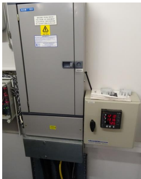
Figure F1: Distribution board with permanent meter located next to it.
