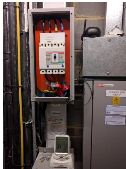
Figure F2: Distribution board with short-term monitoring equipment.
