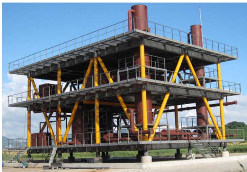
(a) Hypothetical FLNG topside structure at the KOSORI test site
