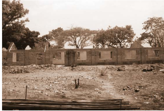
Lainya Vocational Training Institute. Unlike Torit, the original buildings in Lainya were totally destroyed during the war. c. Dr. Dominic Odwa Atari , March 2009.
