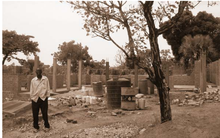
Rebuilding Lainya Vocational Training Institute. c. Dr. Dominic Odwa Atari , March 2009.
