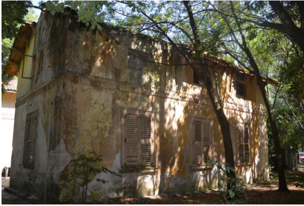
Figure 8 – British rule barracks building, photo: Alexandra – Aikaterini Andrianou, April 2017
