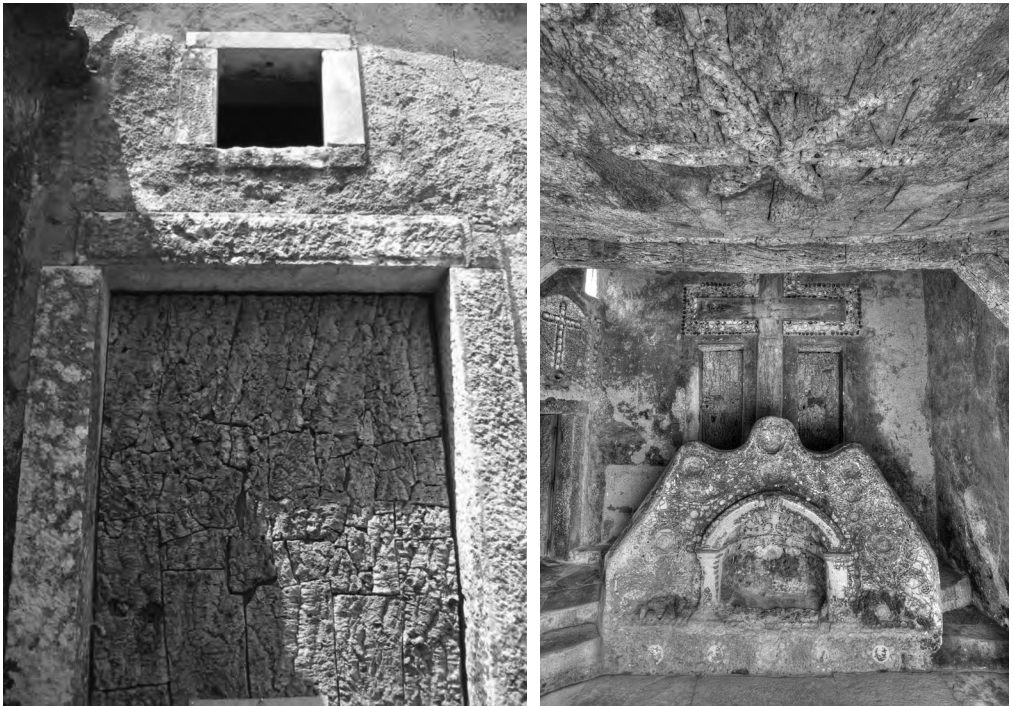
Figure 3. The Convent of the Capuchos, Sintra, Portugal. Left: Cork clad door. Source: Board of Trustees, RBG Kew CC BY 3.0. Right: Interior with ornamental use of cork to ceiling. Source: Parques de Sintra. © PSML-EMIGUS
