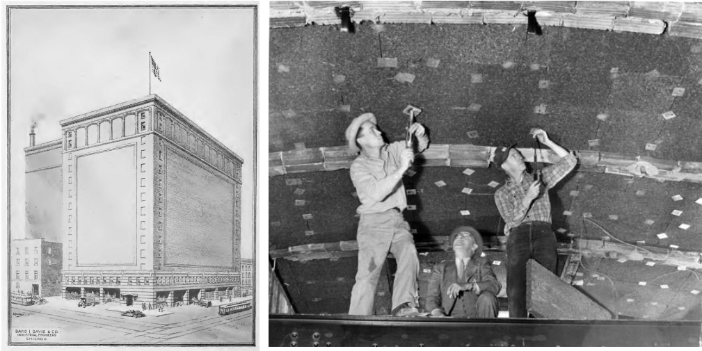
Figure 5. Left: Drawing of the Central Cold Storage Company building, Chicago, 1917, the “Largest Modern Cold Storage Warehouse in the World” at that time.[28]. Right: Workmen installing cork insulation on the White House ceiling during renovation works, with President Truman looking on, Washington, 1951. Source: Abbie Rowe, National Park Service. Harry S. Truman Library & Museum.
