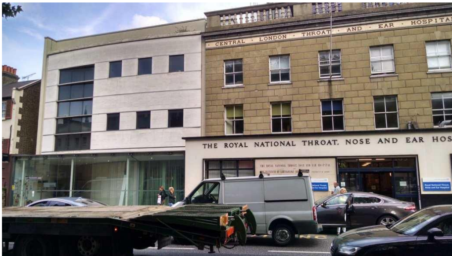
Entrance of the Royal National Throat, Nose and Ear Hospital from across the road
