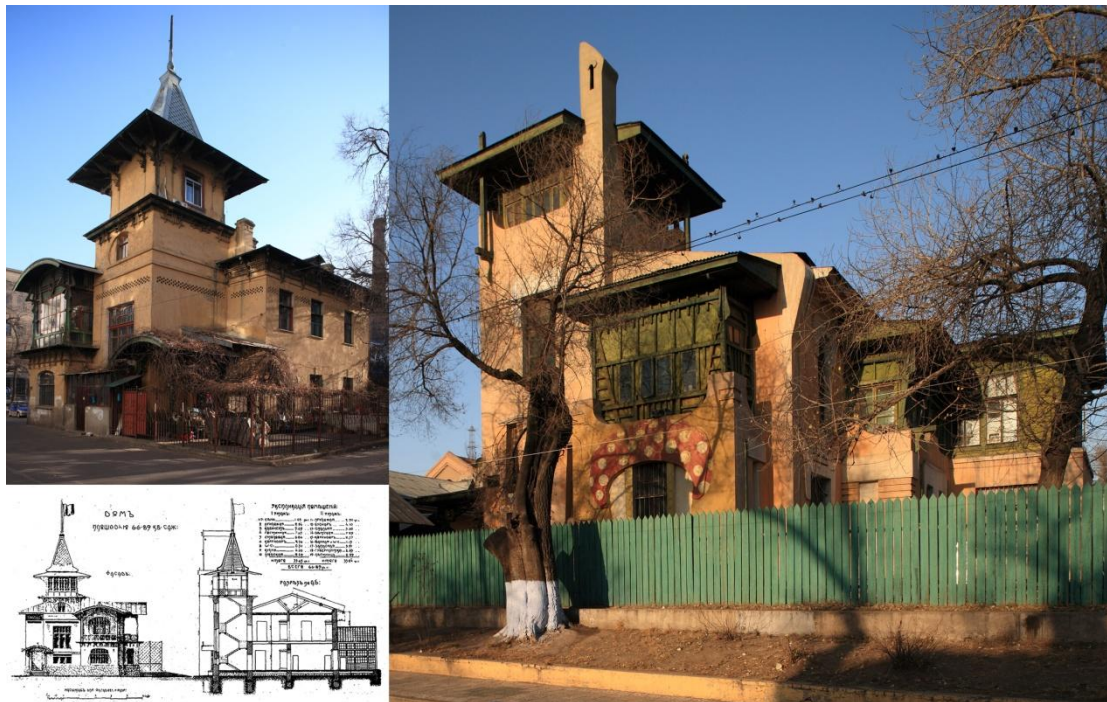
Fig.01: Examples of the many residences for the staff of Russia's China Eastern Railway, designed in the early 1900s in an Art Nouveau style.
