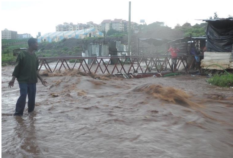
Figure 4. Andolo Bridge flooded at after a 30-minute rain on May 2016. (Photo by Pascal Kipkemboi. Source: Wandera, 2016).
