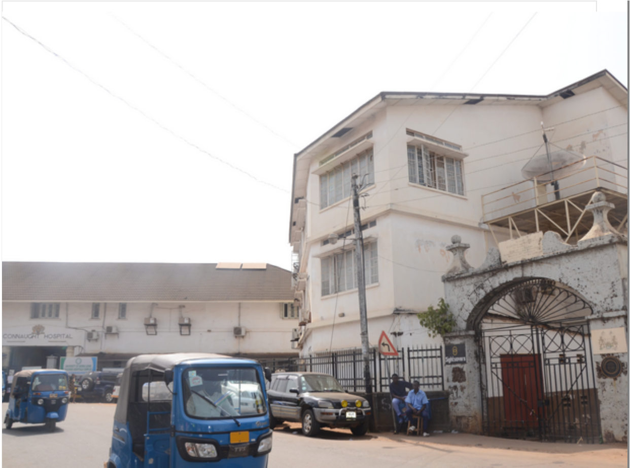
Fig. 1 Connaught Hospital and King's Yard Gate. Source: Photography by author.
