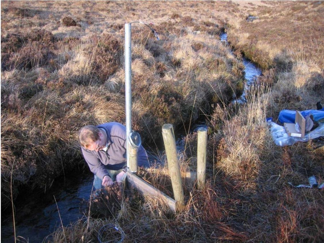
Figure 13. Installation of stilling pipe, 19<sup>th</sup> January 2011 at the Round Loch of Glenhead outflow (Photo Chris Curtis).
