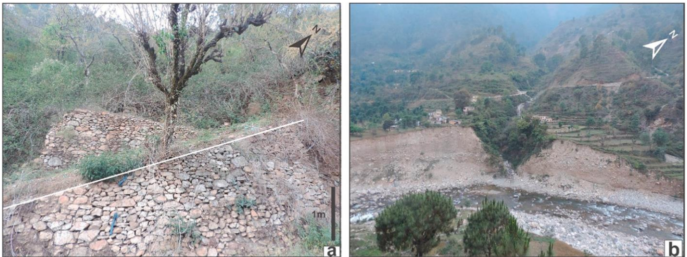
Fig. 14. (a) Tilted Tree and retaining walls show recent activity along stabilized landslide material (b) River toe cutting near Lata village along Balganga valley.
