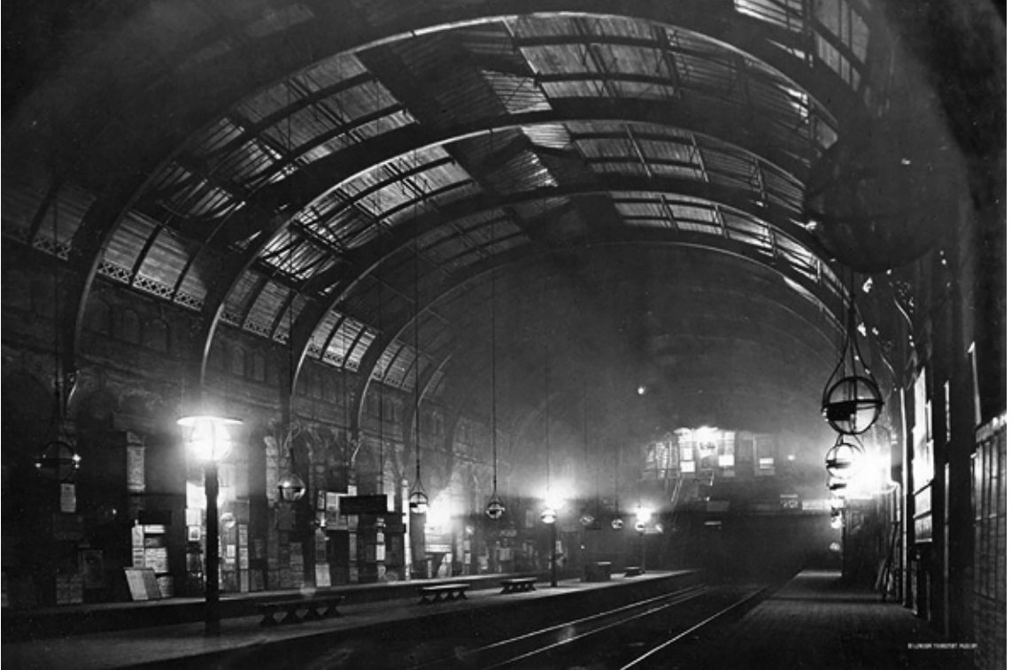
Figure 4: Aldersgate Street station, photographed by Henry Dixon on 22 April 1880, showing electric lighting installed in August 1879, including lampposts supporting spherical lamps along the central island platform, supplemented by wall mounted lamps hanging above the side platforms. London Transport Museum: Inventory number 1998/84029.
