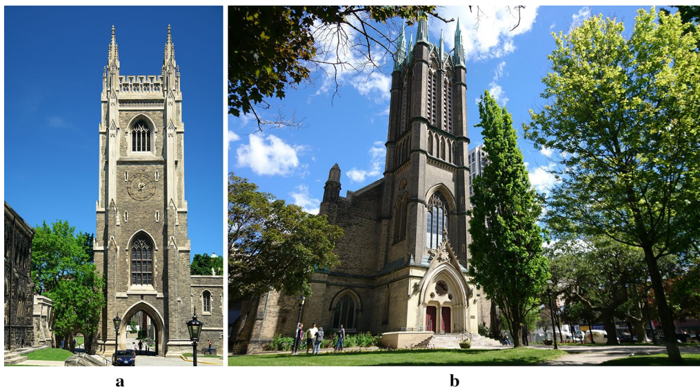
Fig. 2 External façades of the two carillon towers investigated. a Soldiers' Tower that houses the carillon, as seen from Hart House Circle. "Soldiers' Tower 2007" by V. Samarin is licensed under CC BY 3.0 ( https://commons.wikimedia.org/wiki/File:Soldiers_Tower_2007.jpg ). b The carillon tower of Metropolitan United Church, as seen from Queen St E
