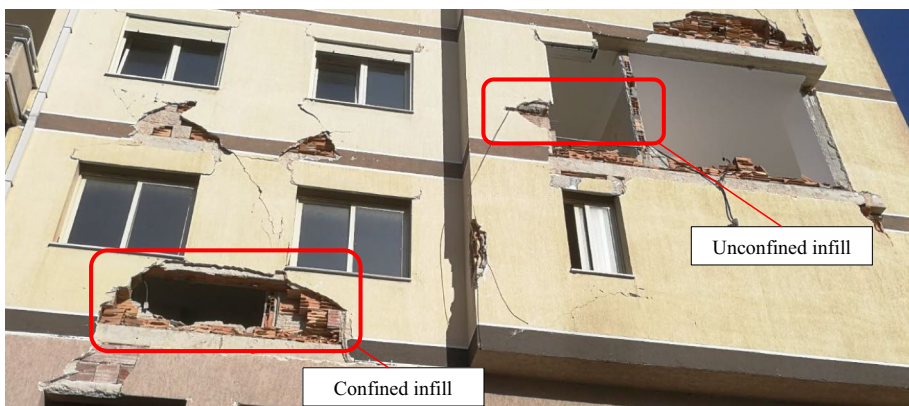
Fig. 14 Typical 2010+ multi-storey reinforced concrete (RC) building compliant with KTP-N.2-89 with integration based on the Eurocode 8. Effects of the belt beams in confined and unconfined infills
