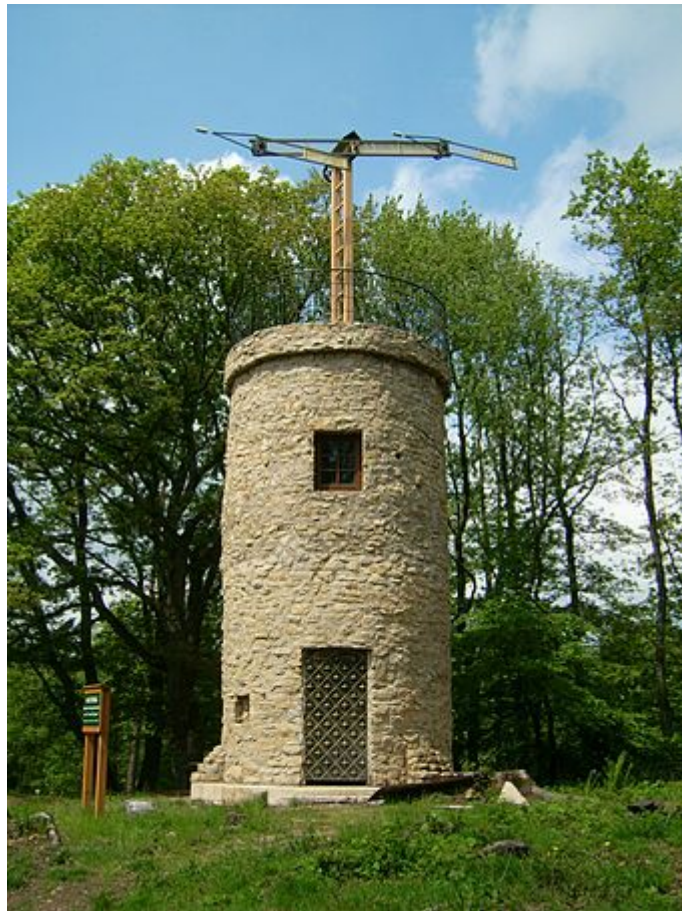
Figure 2: A replica of one of Chappe's semaphore towers in Nalbach, Germany
