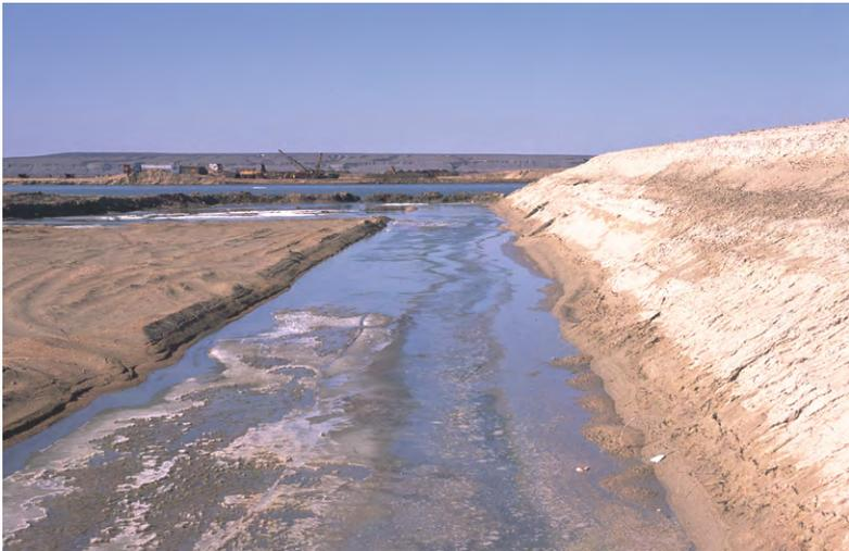
**Figure 5.9** Kökoral dyke under construction, 2004. Southern slope of dyke. The dam and sluice gates have yet to be installed. The cliffs of the former Kökoral island are visible in the background. Photograph by Vincent Robinot.
