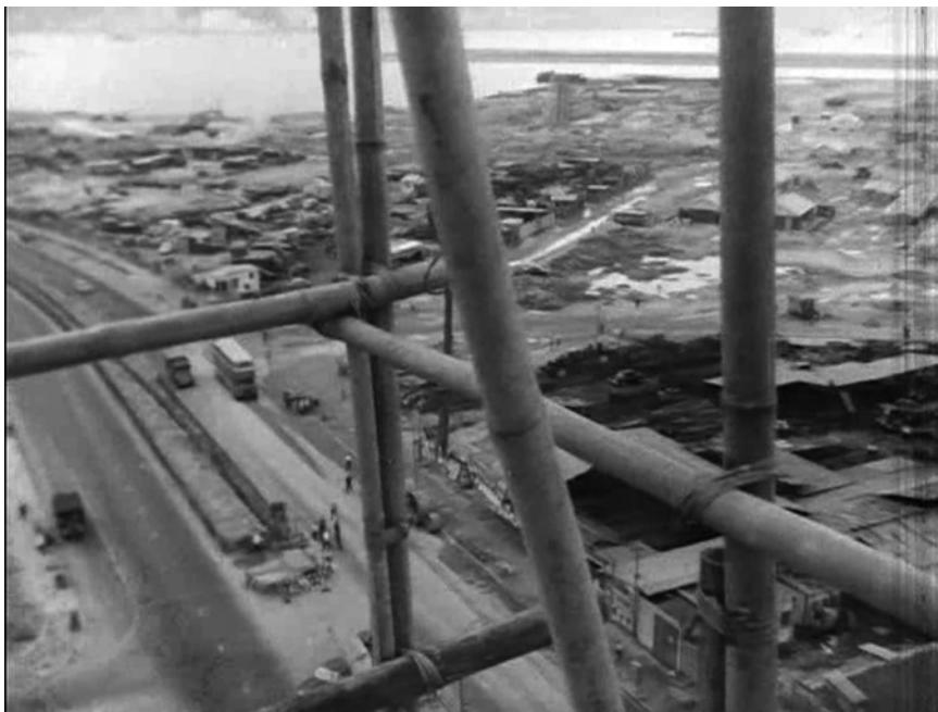
Fig. 7: Surveying the squatter settlement in Discharged Prisoner
