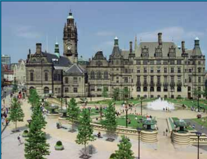
Sheffield Town Hall and the newly redesigned Peace Gardens – a flagship and award-winning project in the regenerated heart of the City.
