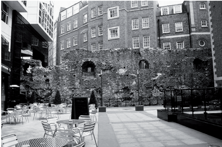
Figure 3. City Wall, Cooper's Row, London (Photo by C. Sandes).
