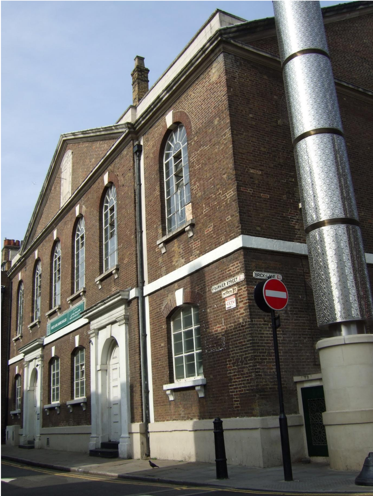
Figure 7: Jamme Masjid minaret and mosque, Brick Lane.
