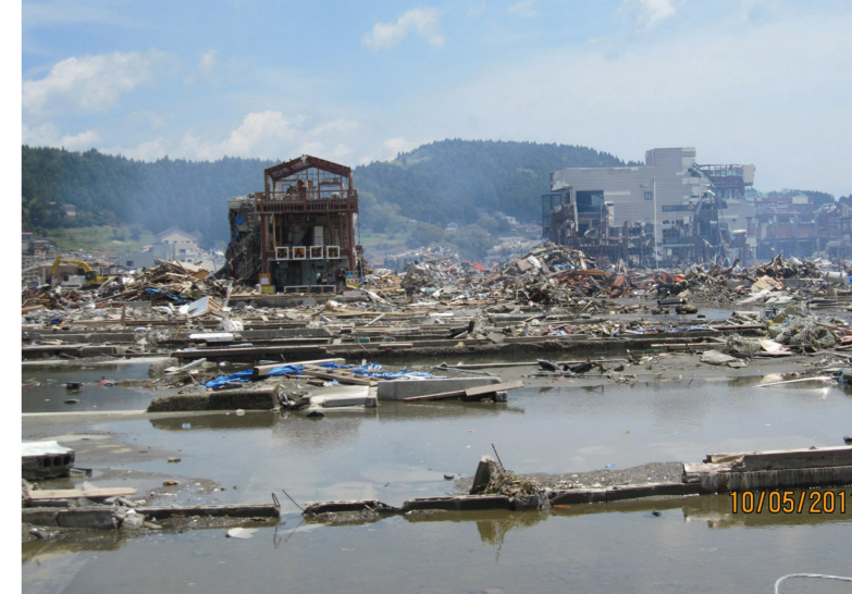
► Extensive tsunami damage at Manamisanriku following the Tohoku earthquake and tsunami on 11 March 2011. Photograph courtesy of David Tappin of the British Geological Survey and taken on 10 May 2011.
