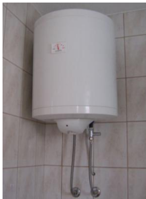
Figure D2.1 An example of installed electric heated domestic storage water heater
