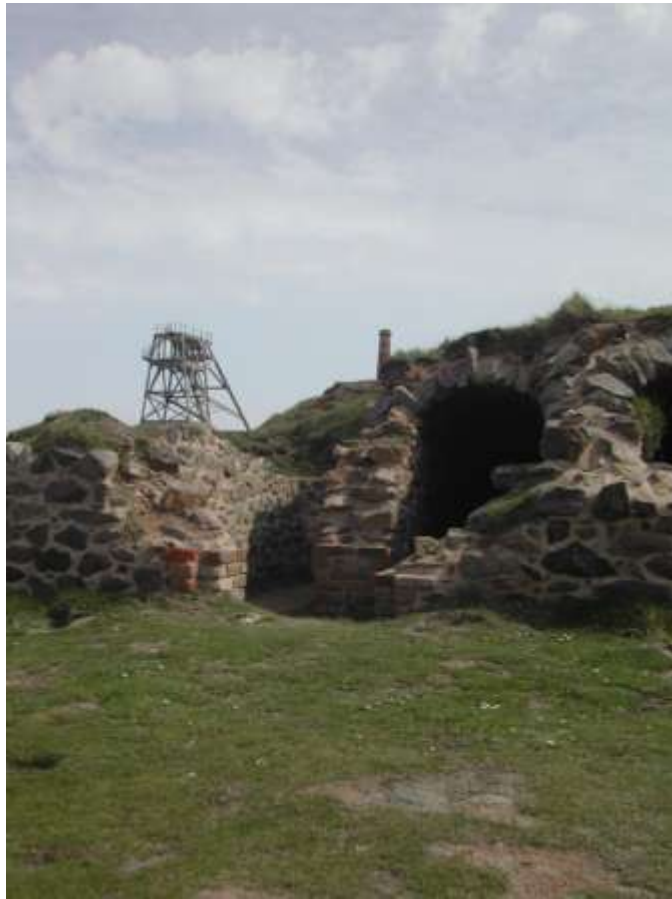
Figure 7.5 Arsenic labyrinth with headframe of Allen's shaft in the background. Photo © Hilary Orange
