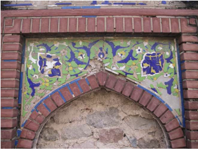
Fig. 3. A mosaic composition of glazed tiles on the wall mosque at Atgah Khan's Tomb.
