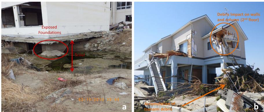
**Fig. 8** **a** Severe scour caused by the 2011 tsunami, exposing the buildings foundations (structural damage, at least DS4); **b** extensive damage mainly due to debris impact on the second floor (*wood*), structural damage. **a** Courtesy of Dr J. Bricker, Tohoku University
