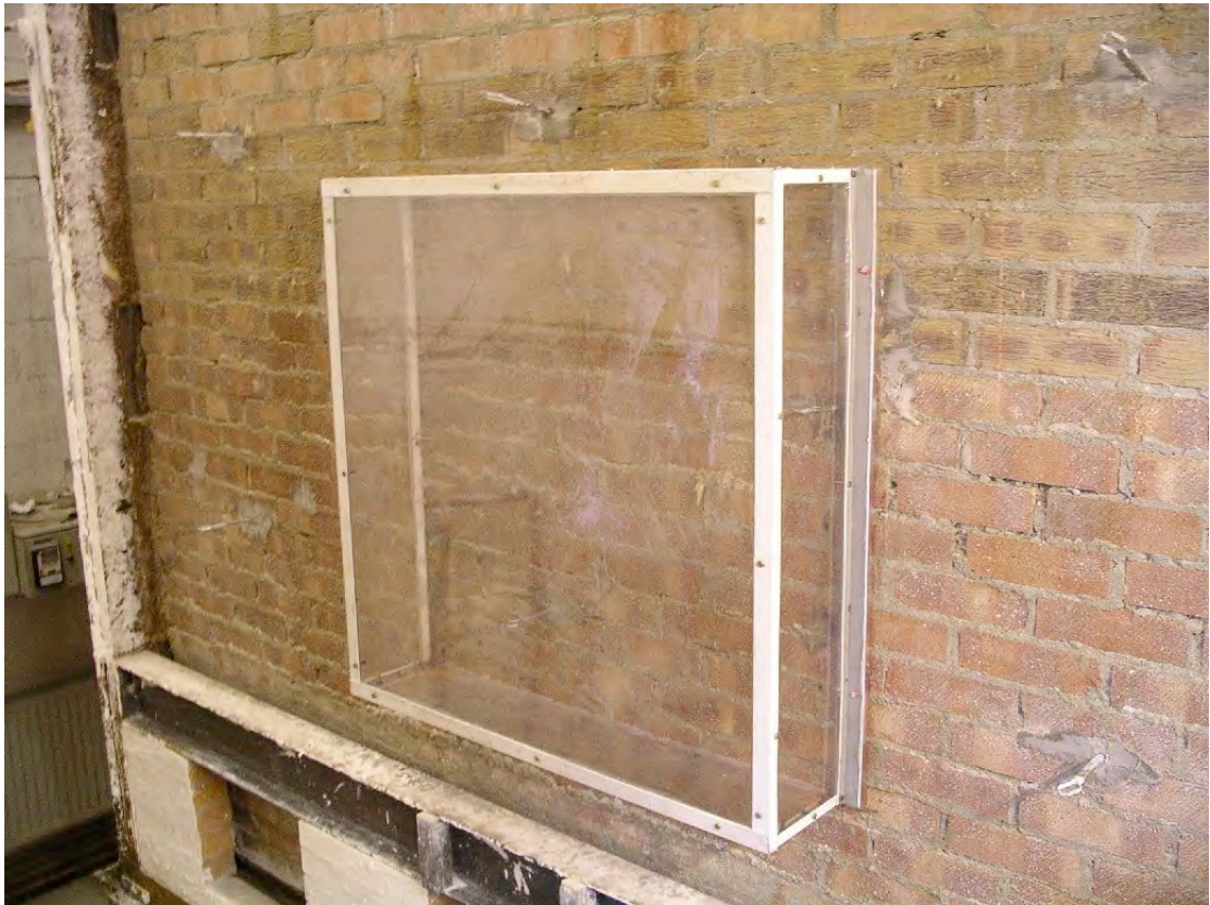
Figure 3.5, Perspex box attached to brickwork
