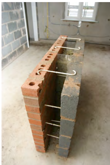
Figure 1.0, A 142mm cavity (yet to be filled) that could satisfy future thermal performance demands. This width of cavity was used in a trial on a recently built housing estate in the north of England.
