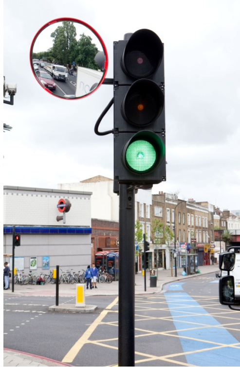
Figure 37: convex mirror situated adjacent to traffic signals (TfL image)
