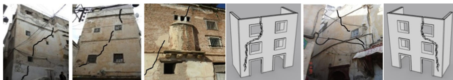
Fig. 11 In plane mechanism
