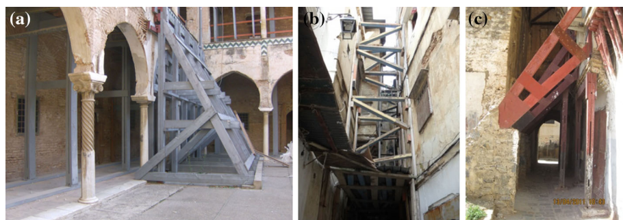
Fig. 17 a Shoring system made of wooden trusses used to prevent out of plane failure of masonry walls in The Casbah of Algiers, b shoring system applied to buildings facing a narrow street and c system of shoring also supporting the q'bu
