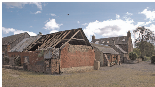
Figure 6. Flatfield Steading, with the instrumented western gable end of the barn building in the foreground
