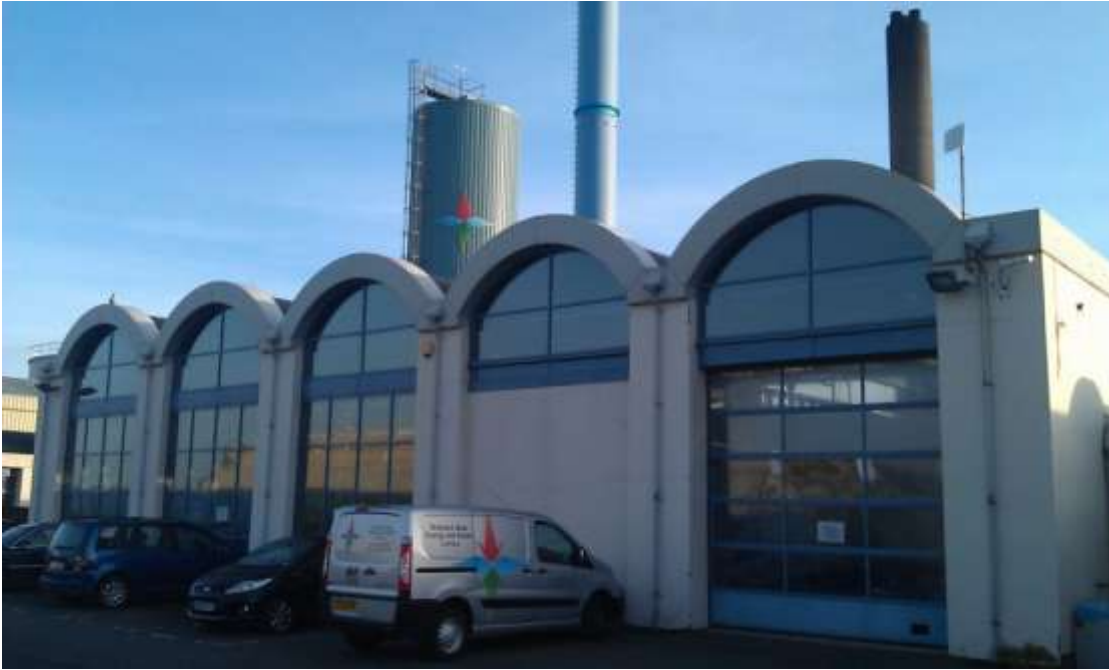
Figure 17: Photograph of the central pumping station for Shetland Heat and Power Limited (Cary, 2011)
