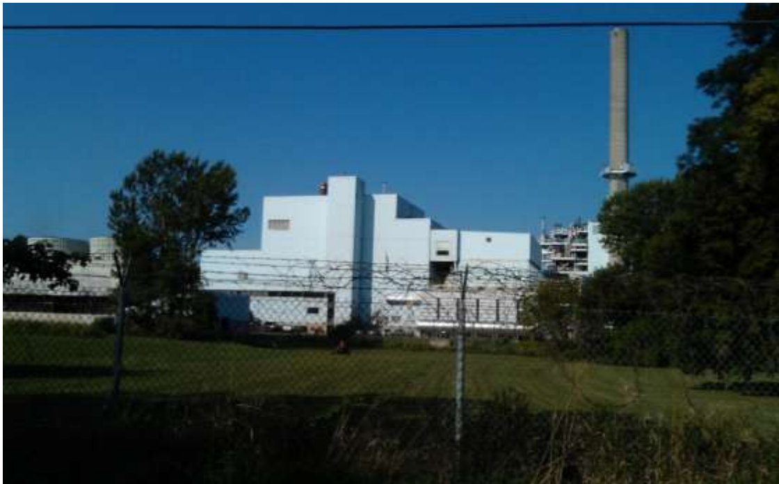
Figure 12: Photograph of McNeil Generating Station (Cary, 2012)
