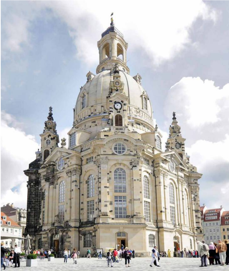
FIGURE 2 The rebuilt Frauenkirch showing the surviving sections and reused material in darker colours.
