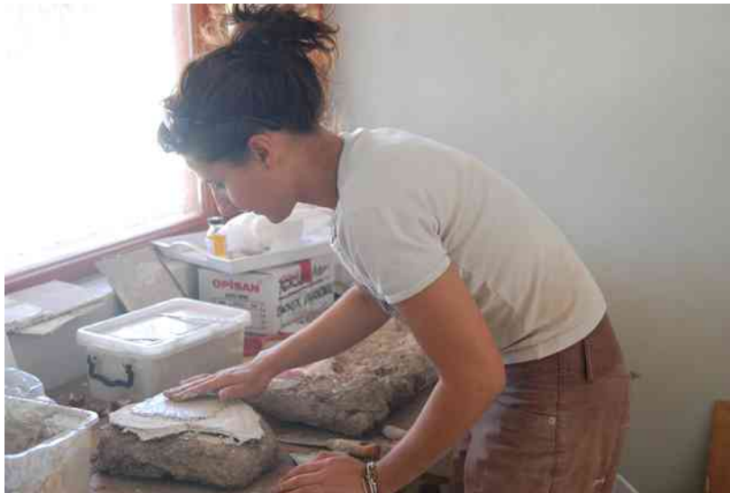
Fig.144 Smoothing out marl plaster by hand.
