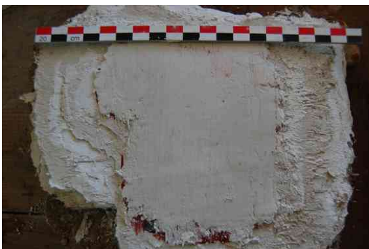
Fig.157 A thin layer of marl plaster applied over a painted layer.
