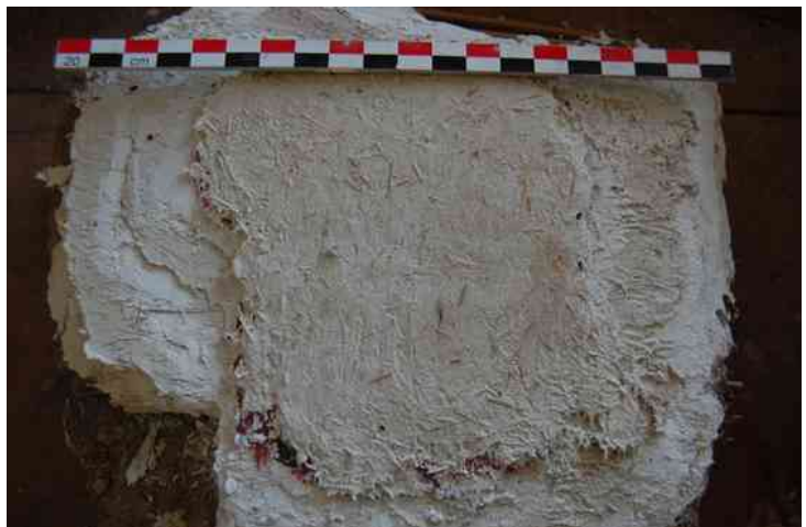
Fig.159 Pale brown marl plaster layer mixed with plant inclusions creating a thicker layer to cover the paint layer below.
