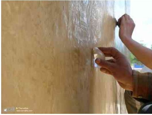
Fig.161a Polishing Tierrafino plaster with small hand held semi-precious stones ( www.tierrafino.com/stone_tadelakt_gallery/material%20and%20workshops/ ).
