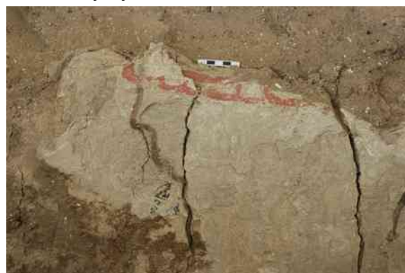
Fig.29 A wall painting from 4040 Area, U.12314, Sp.256 showing cracking (Jason Quinlan, Çatalhöyük Research Project)
