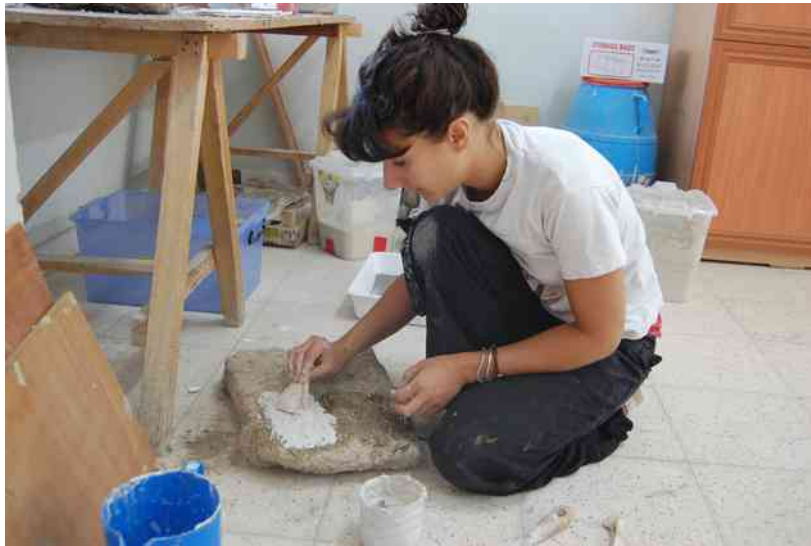
Fig.143b Spreading marl plaster onto mudbrick using a small sheep scapula.
