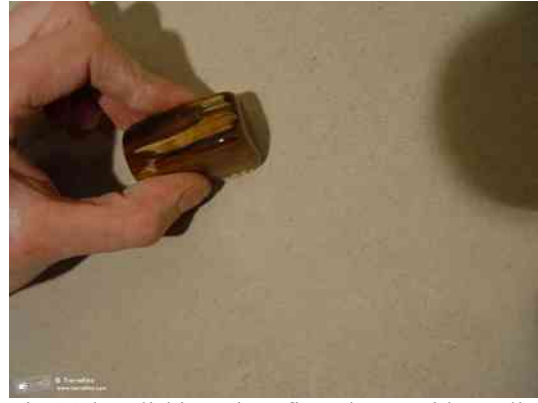
Fig.161b Polishing Tierrafino plaster with small hand held stones ( www.tierrafino.com/stone_tadelakt_gallery/material%20and%20workshops/ ).
