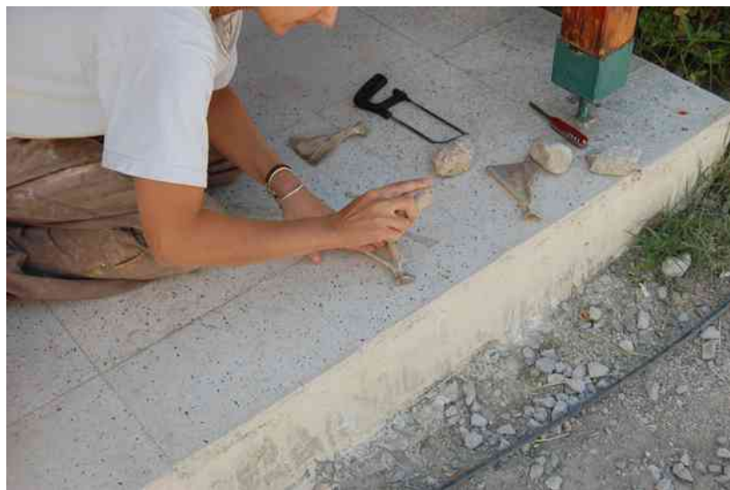
Fig.143a Working the sheep scapulae into shape before plastering.
