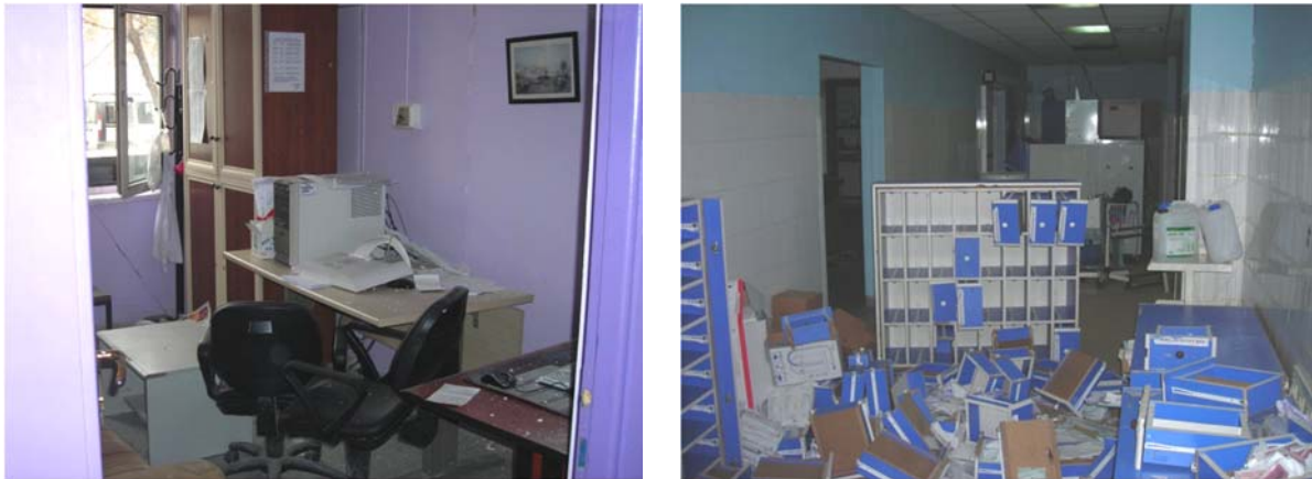
Figure 2. Damage to the building contents surveyed in the aftermath of the 2011 Van (Turkey) earthquake in the Yüzüncü Yil University – Faculty of Medicine Hospital.
