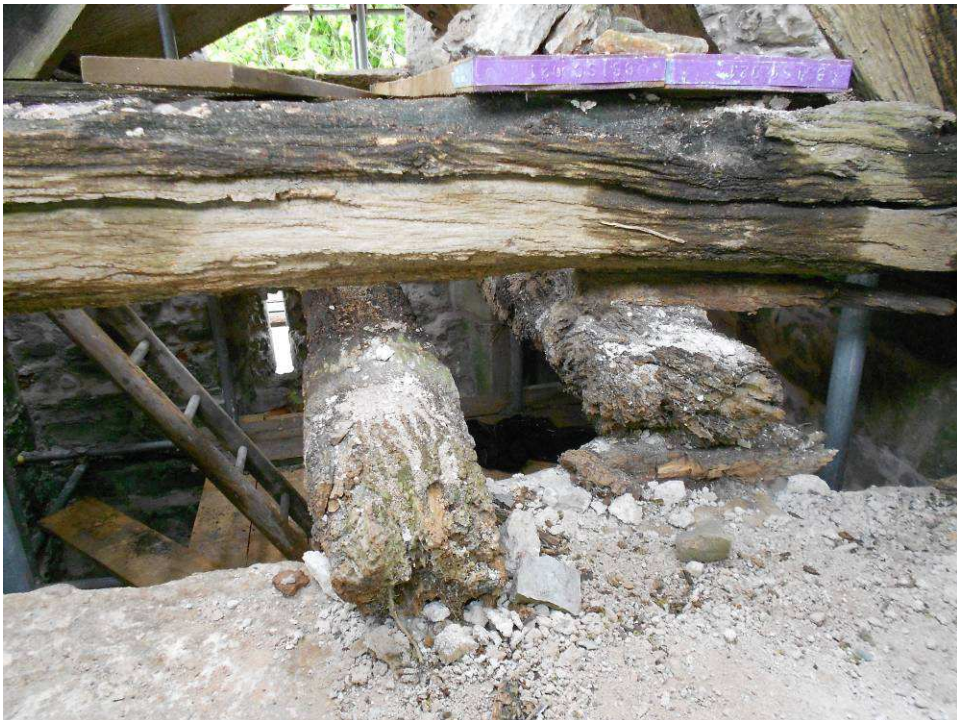
Figure 4: Two of the support beams to the bell frame (Tim Allen)
