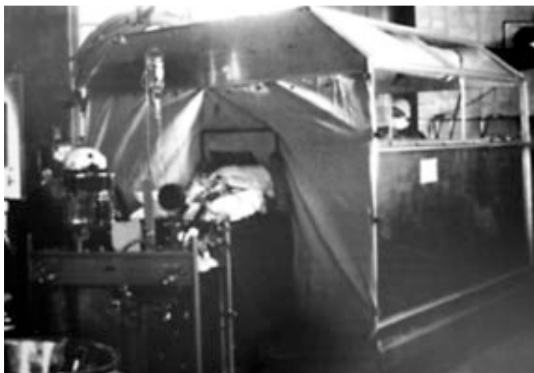
Figure 12: Charnley's original greenhouse clean air enclosure, 1960.
