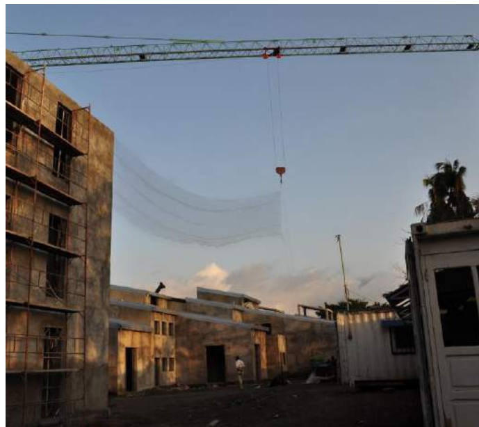
Figure S2.12 Location of mist net for catching E. helvum bats in Malabo Bioko, demonstrating that this species appears content to roost in highly urban environments, and the successful and novel use of a construction crane to set mist nets.
