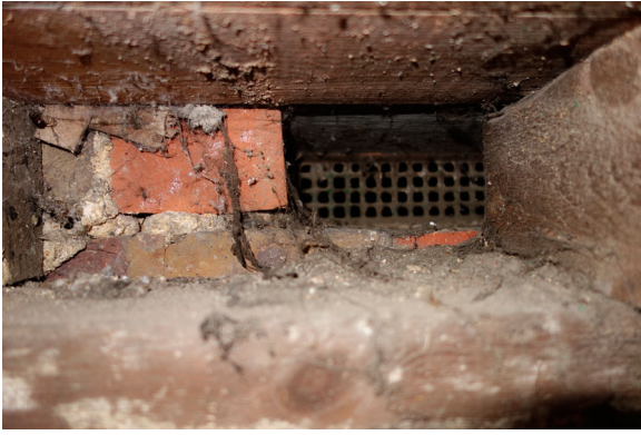
Figure 2. An airbrick in between the joists.
