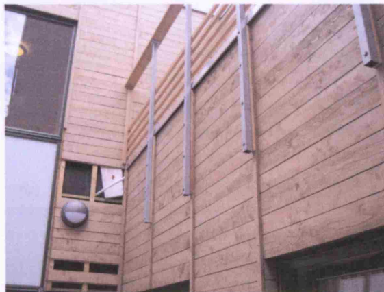
Fig. 14: Use of Douglas fir as external wall covering
