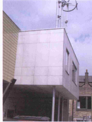
Fig. 18: Use of aluminium sheets as wall cladding
