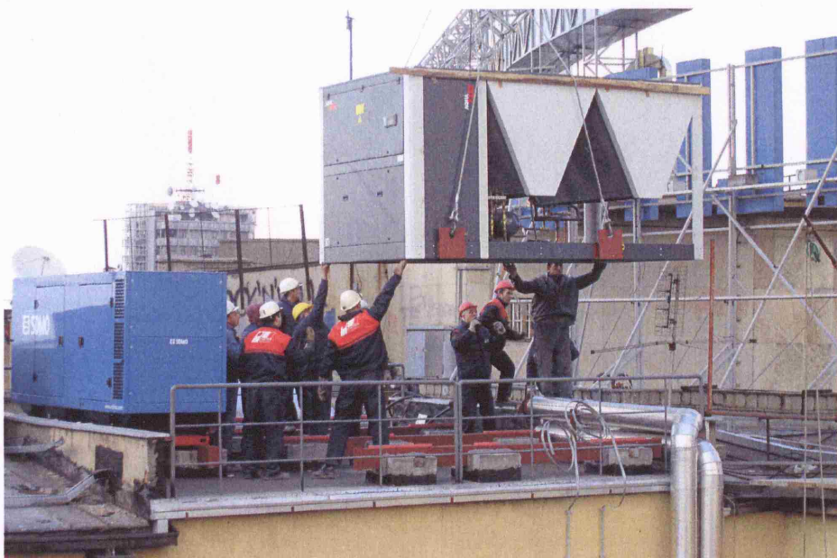
Fig.17. -Air handling unit of the auditorium located on the roof
