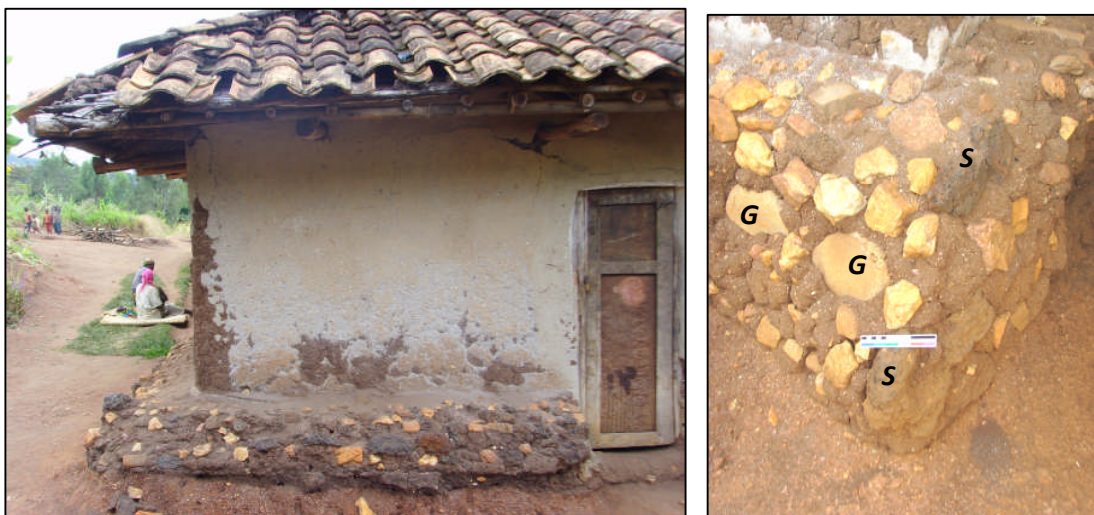
Fig.6.5.4 House foundations at KMA constructed with small, layered slag blocks (S), and grinding stones (G)
