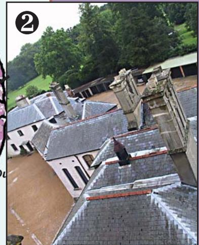
2. The complex roofs of historic houses make them especially vulnerable to wind damage. Damaged roofs and rainwater goods are followed by water ingress, causing severe long-term problems to the historic fabric and interiors.
