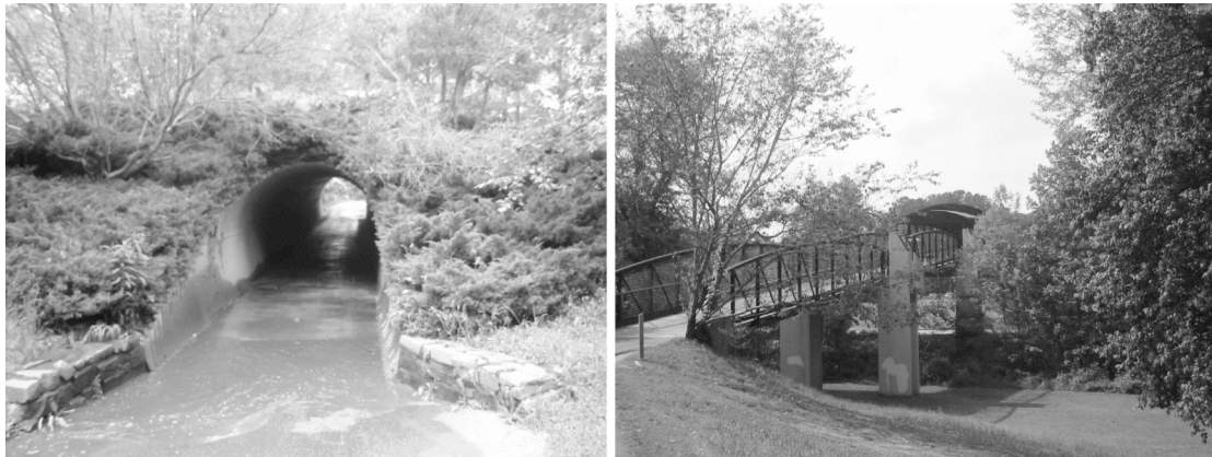
Figure 3. View of a Typical Cart Path Tunnel and Bridge Crossing
